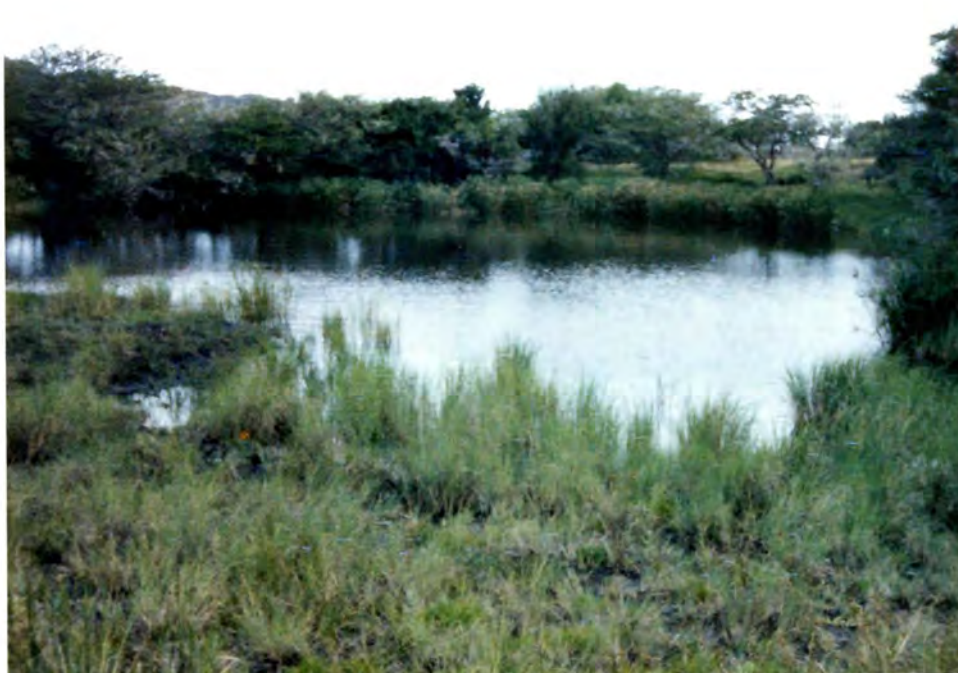
Fig. 10. A general view of Rufanes Pool. The dam wall is on the left side of the photograph.
