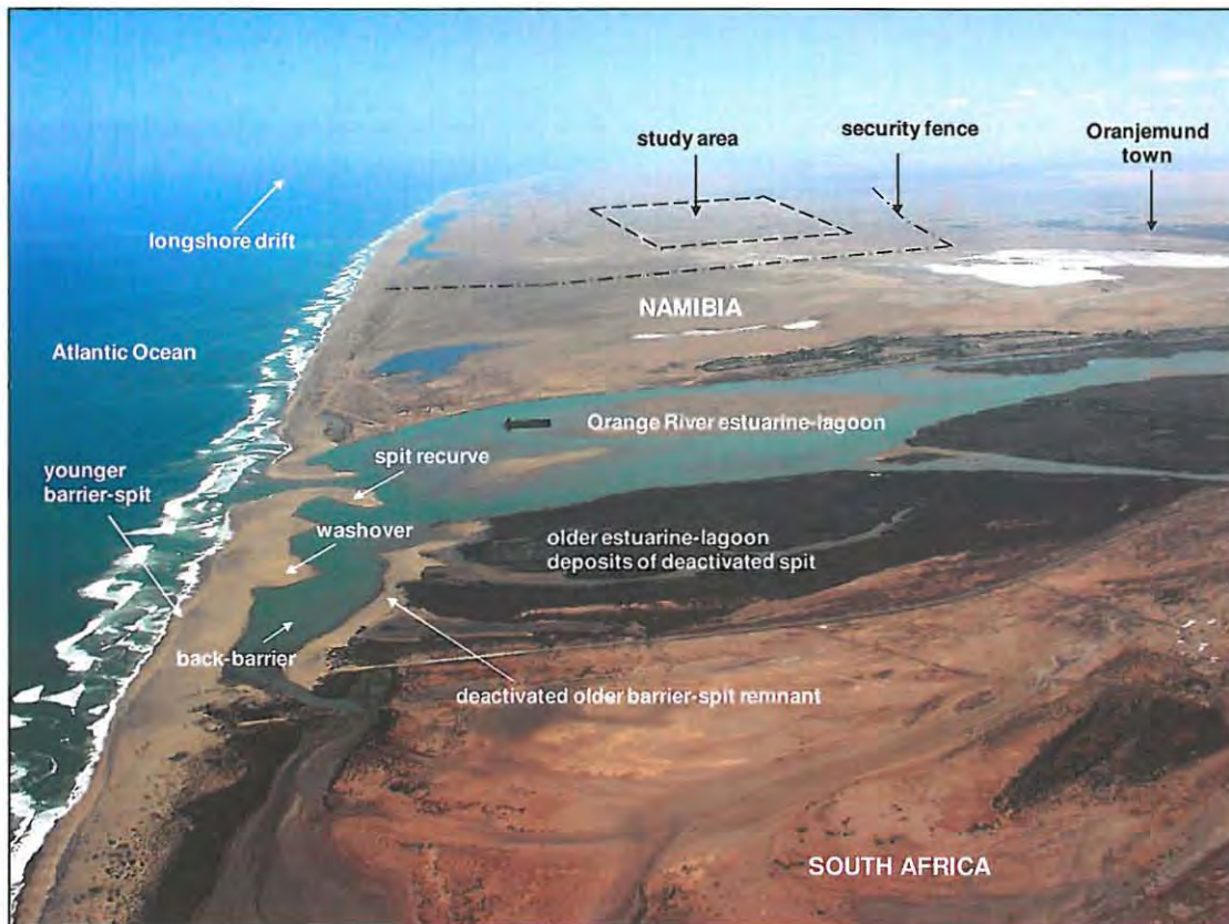
Figure 4.7: Modern example of a deactivated barrier in Oranjemund, Namibia. Oblique aerial view (2003) of the present Orange River mouth setting, looking northwards towards the study area. A deactivated barrier, now an abandoned remnant, is positioned landward and protected from the wave energy by a younger, active barrier feature. Note that current sea-level along the west coast of South Africa and the Namibian coast is rising (see Hughes et al. , 1991) and thus the shoreline depicted in the aerial photograph is an expression of a transgressive system, which is also evidenced from the washover deposits. A similar setting of barrier abandonment and isolation is envisaged for the study area. Solid black arrow in photograph depicts river flow direction. For measure of scale, length of de-activated barrier is approximately 700 m.
