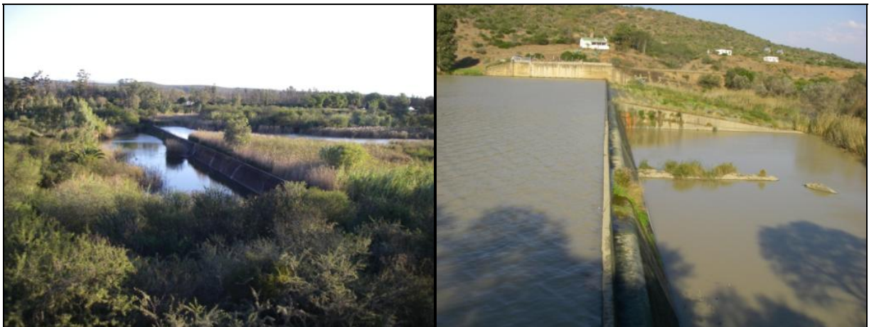
Figure 6.3. Cleveland weir (left) and Korhaansdrift Dam (right) on the Sundays River (photographs courtesy of Olaf Weyl)
