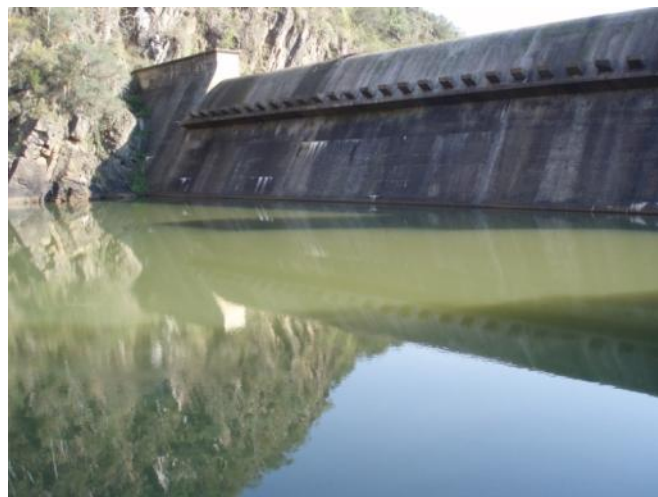
Figure 6.7. Slagboom Dam wall on the Wit River, a partial barrier to upstream eel migration, and a complete barrier to the upstream migration of other fish species
