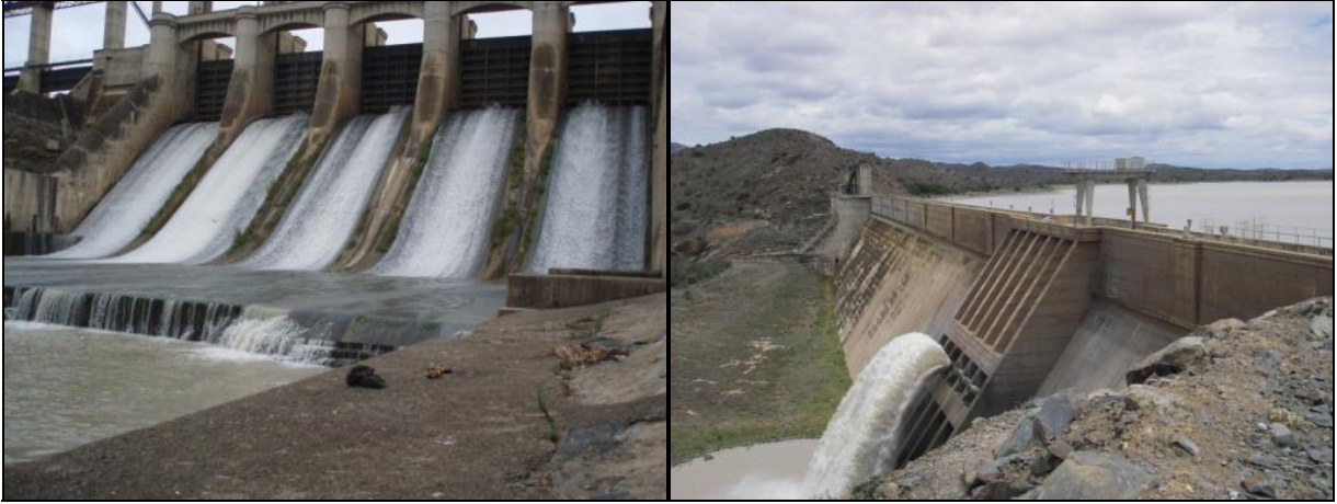
Figure 6.4. The 48 m high Darlington Dam wall, with 5 spillways (left) and six main outlet valves (right). (right photograph courtesy of Olaf Weyl)
