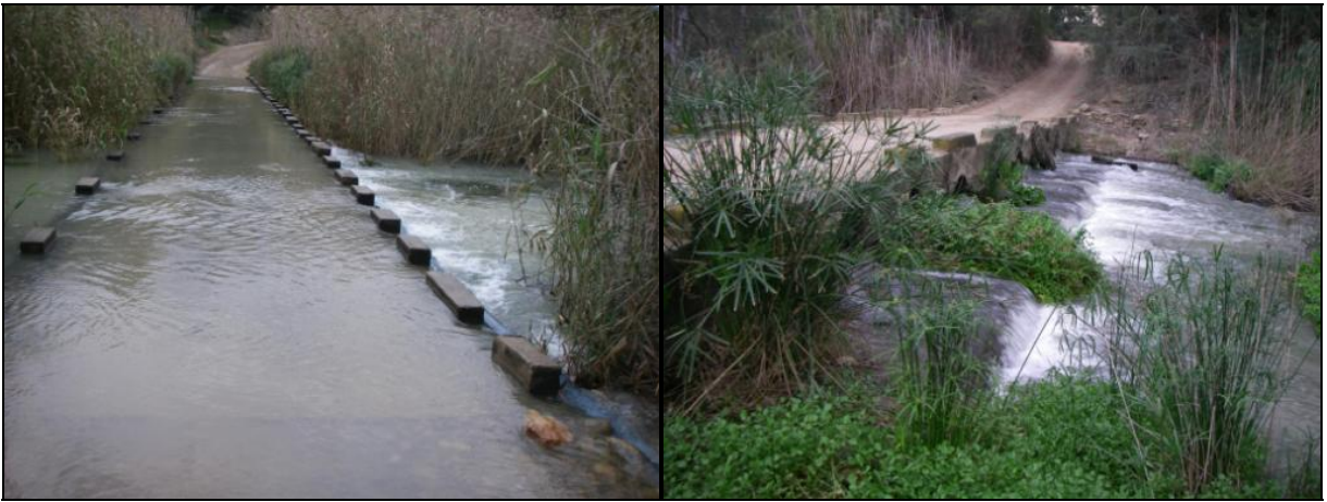
Figure 6.5. Two of the six causeways on the Sundays River that are partial barriers to the upstream migration of fish (photographs courtesy of Olaf Weyl)
