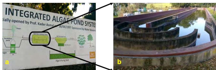
Figure 1. 1 Integrated algal pond system (IAPS) located at EBRU experimental station, Makhanda District, Eastern Cape Province, South Africa. Flow and outcome design (a), high-rate algal oxidation pond (HRAOP) containing microalgae-bacterial flocs (MaB-flocs) as sources of environmental samples (b).
