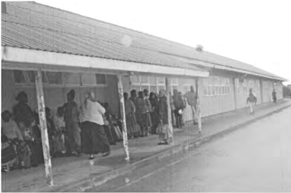
Fig. 3. Queuing outside the building
