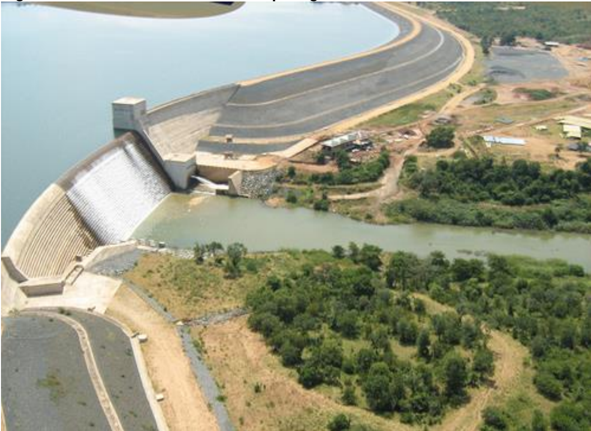
Figure 4.6: The Nandoni Dam over-spilling
