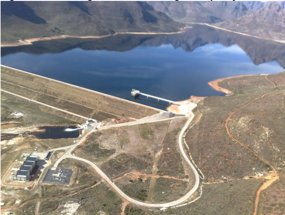
Figure 4.7: The Berg River Dam nearing full capacity
