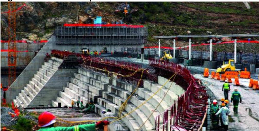
Figure 4.1: The De Hoop Dam under construction
