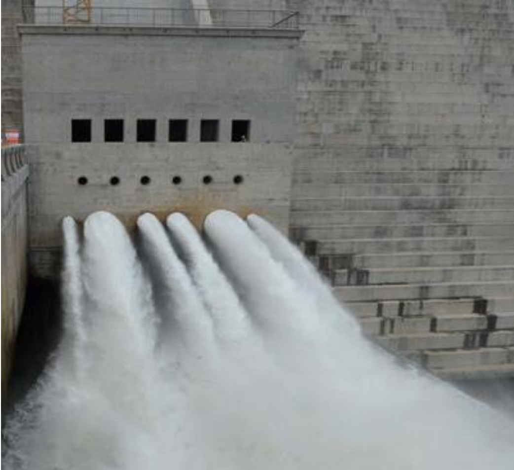
Figure 6.1: Releasing of water from the De Hoop Dam.
