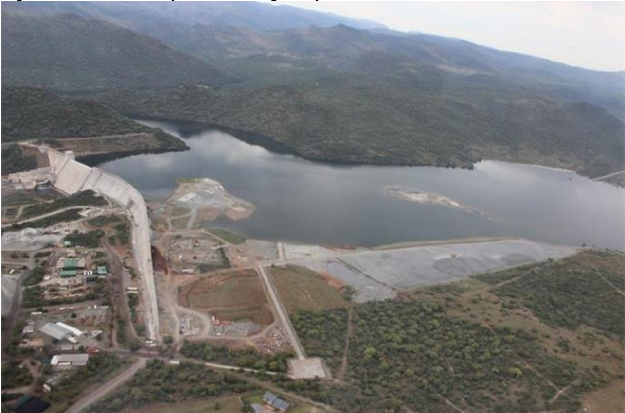
Figure 4.8: The De Hoop Dam nearing completion
