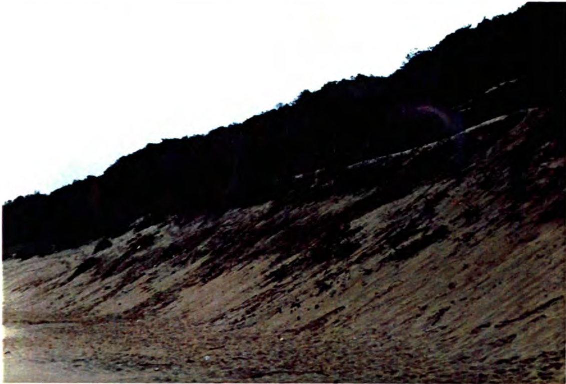
Plate 8.3 Slope failure of the Cintsa Bay stabilization site due to wave attack. The dominant vegetation above the erosion scarp is Chrysanthemoides monilifera .
