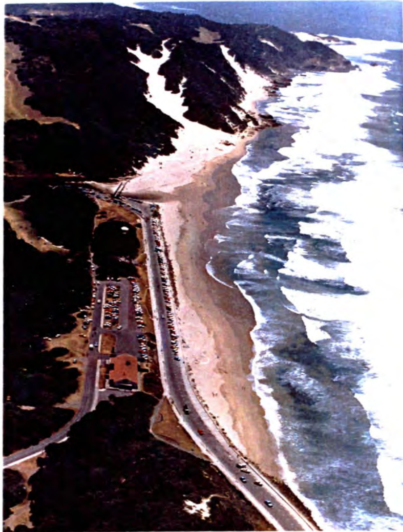
Plate 5.1 Aerial view of the Eastern Beach and Esplanade area looking east towards Nahoon Beach. The large building is the cafe and restaurant, and behind this is the Marina Glen. The road sited in the dynamic zone of the beach is clearly visible.
