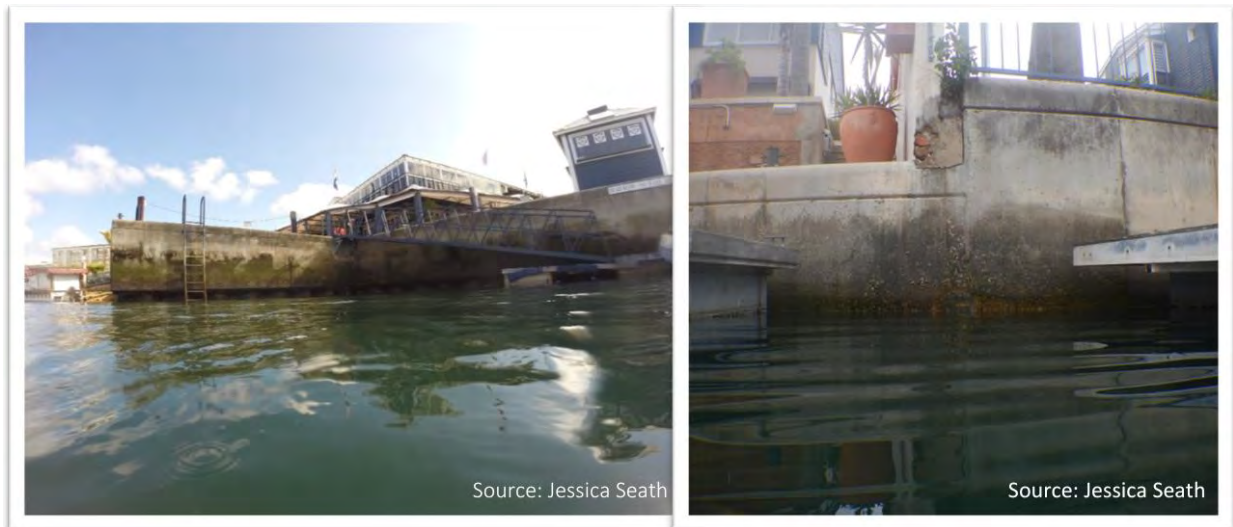
Figure 2.2: Concrete vertical seawalls along the edges of Knysna Harbour within the Knysna Estuary (view from the water).
