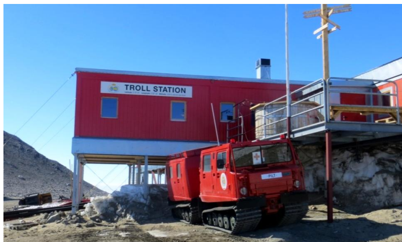
Figure 5b. Troll Station.
