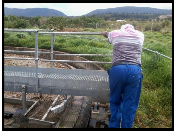
Figure 3.17 Clarifier at the Kirkwood WWTW, October 2012 (left). The automated clarifier sometimes stopped and needed assistance getting moving again (right).
