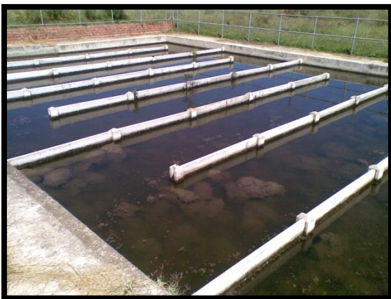
Figure 3.18 Large amounts of sludge in the maturation ponds due to the broken clarifier, October 2012 (left). Suspended sludge exiting the WWTW and heading to the effluent discharge point, October 2012 (right).
