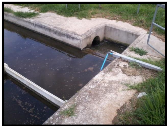
Figure 3.18 Large amounts of sludge in the maturation ponds due to the broken clarifier, October 2012 (left). Suspended sludge exiting the WWTW and heading to the effluent discharge point, October 2012 (right).
