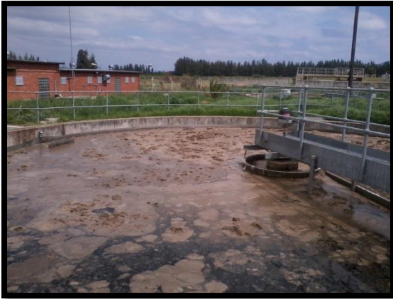
Figure 3.17 Clarifier at the Kirkwood WWTW, October 2012 (left). The automated clarifier sometimes stopped and needed assistance getting moving again (right).
