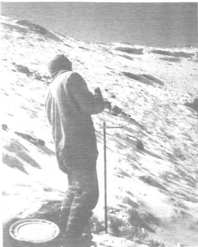
Figure 4.7: Preparation of the ground for polyethylene tube insertion (May 1995).
