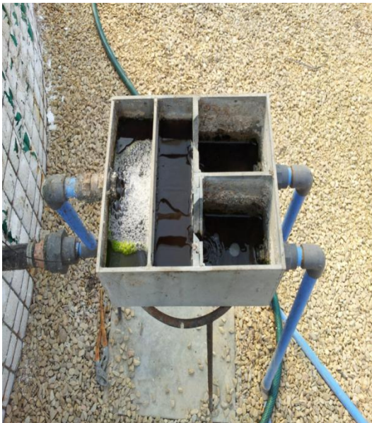
Figure 3.5 The splitter box splitted primary facultative pond (PFP) effluent into two streams and directed the effluent into train A and train B of the high rate algal ponds (HRAPs).
