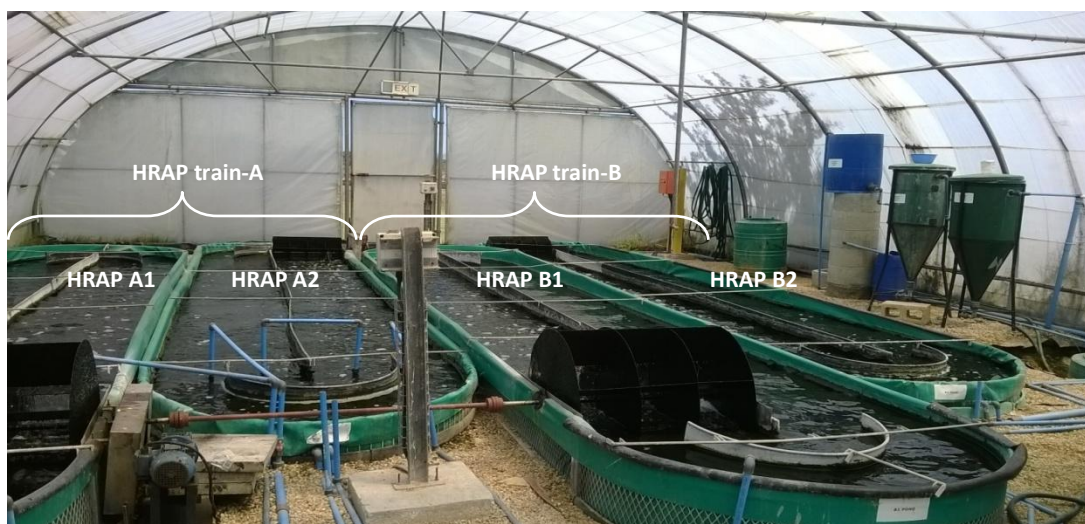
Figure 3.6.a The high rate algal ponds (HRAP) consisted of two parallel trains, each train included two ponds run in series where the numbers 1 and 2 represented the first and second ponds in system A and B respectively. The two algal settling cones and the 500 L pump allowed the recovery of algal biomass.
