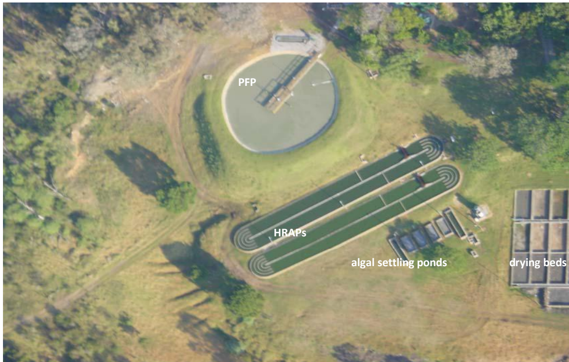
Figure 2.1 An integrated algal ponding system (IAPS) composed of primary facultative pond (PFP), high rate algal ponds (HRAPs), algal settling ponds and drying beds at the Institute for Environmental Biotechnology, Rhodes University (EBRU) for sewage treatment at an experimental scale (Wells 2005).
