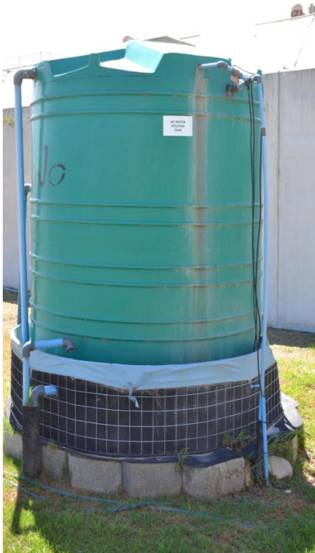
Figure 3.2 The 5000 L anaerobic buffer tank.
