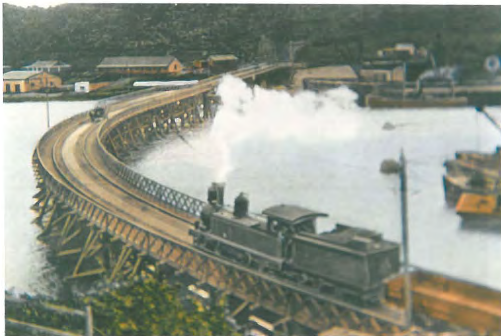
THE "TEMPORARY-PERMANENT" BRIDGE OVER THE BUFFALO RIVER: The so-called temporary bridge was largely a failure in terms of providing a better service for the West Bank. The structure was simply too narrow to accommodate both trains and carriages simultaneously, thereby causing congestion when trains were shunting. As a result, the West Bank would remain a backwater for a further three decades. [Source: East London Museum.]
