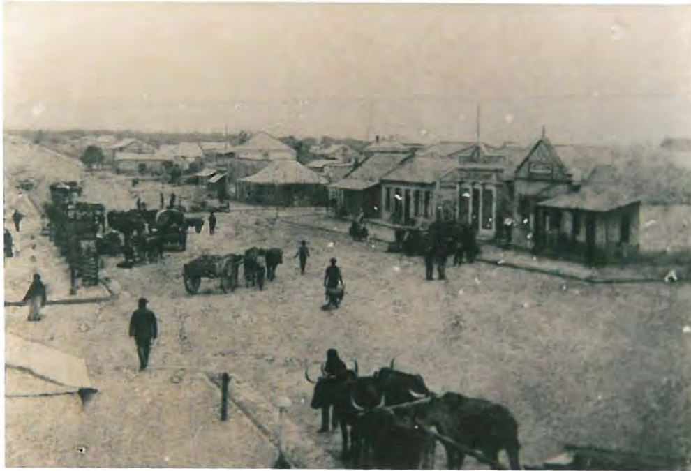
OXFORD STREET IN THE 1880's : One of the earliest photographs of Oxford Street shows a macadamised thoroughfare, with gutters and pavements (the work of the 1881-1882 boom period) but almost no street-lamps. There are also no double-storey buildings which would appear during the prosperous 1890's. [Source: East London Museum.]
