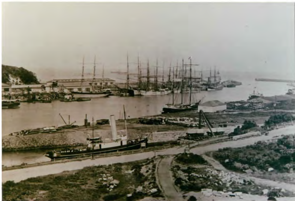
A HAVEN FOR SAILING SHIPS: A notable feature of the increased depth was the fact that the tug (foreground) could accompany sailing vessels into the harbour whereas, previously, it was generally regarded as unsafe to attempt the entry because adverse winds would berth them on the sand-bar or on the rocks. [Source: East London Museum.]
