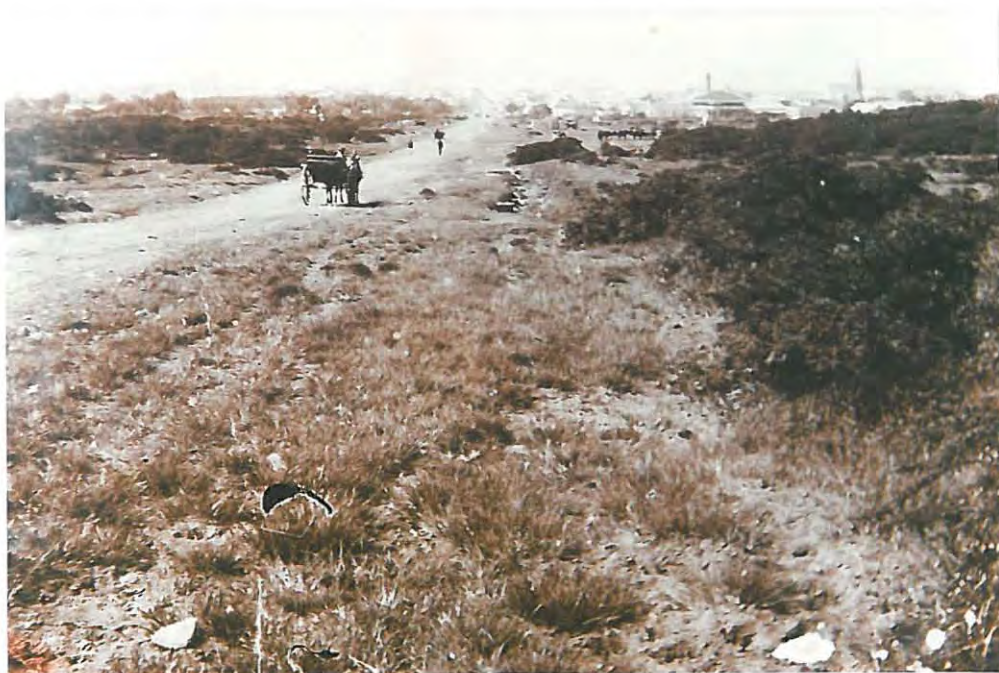
THE STRAIGHTENING OF OXFORD STREET : The last construction work before the "Great Depression" struck was the straightening out of Oxford Street to form a line from the commercial centre of the town to the "Southernwood" acre lots (directly to the left of the camera and out of sight). This picture looks south down the recently "formed" Oxford Street from about the position of today's Medical Centre in St James Road. [Source: East London Museum.]
