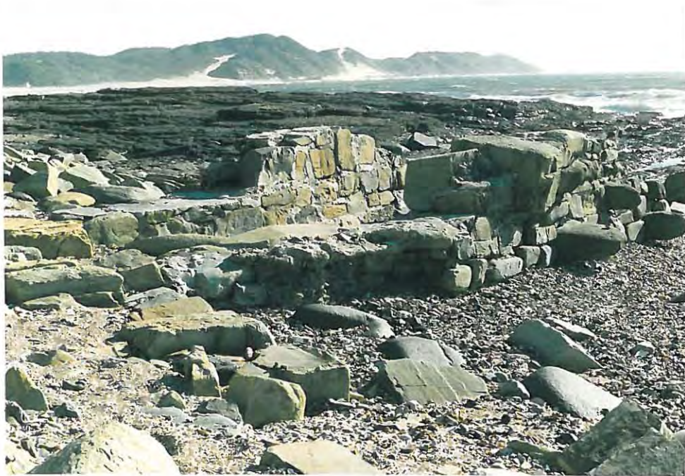
RUINS OF THE BEACH POOL: All that remains of East London's first swimming pool is this double rock wall, a rubble of concrete on the sand and a part of the foundation running in a line towards the sea. The situation of the ruins makes it clear that the Beach Pool was indeed too far away from the sea to be an effective tidal pool.
