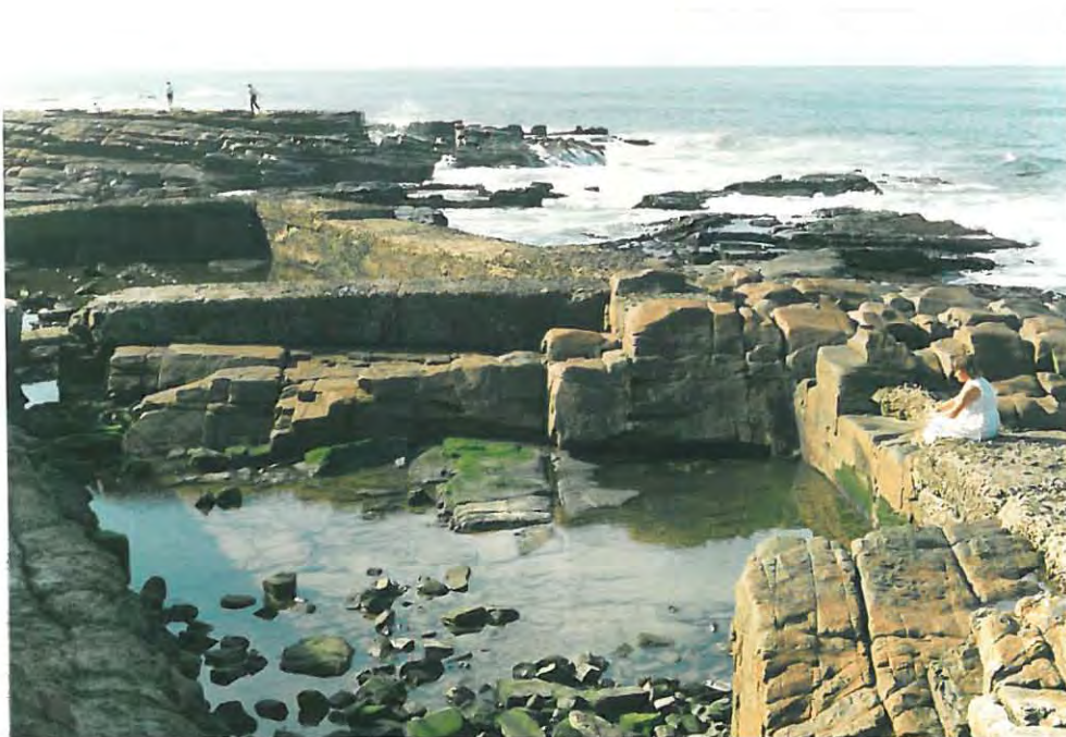
RUINS OF THE QUANZA POOL: Even the popular Guanza Pool had eventually to make way for the much larger Orient Pool. The ruins shown here, however, indicate that the lower end of the pool was close enough to the sea to receive the brunt of the high tides, thereby ensuring that the water remained clean.
