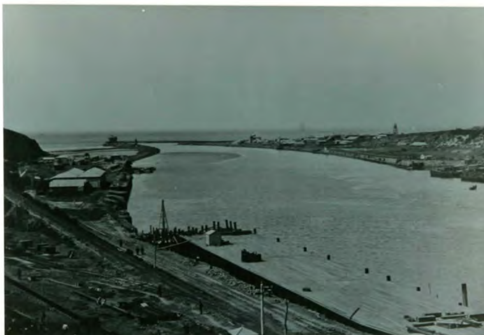
WHARF UNDER CONSTRUCTION (about 1876): The second wharf is built on the east bank of the river. Note that the sand-bar near the mouth partially obstructs the entrance to the harbour, making a channel so shallow that practically no ships can yet enter. Most cargo is still off-loaded in the roadstead on to lighters which are then brought into the harbour by means of tugs. [ Source: Cape Archives, AG 1445.]
