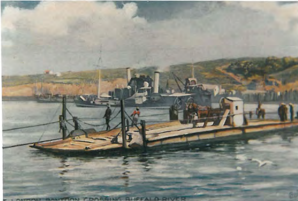
PONTON CROSSING: For a period of five decades the Pontoon remained the only means for wagons, animals and large parcels to be taken across the Buffalo River. The result was the almost complete stagnation of the original village on the West Bank which could not hope to compete with the better endowed East Bank. [Source: East London Museum.]
