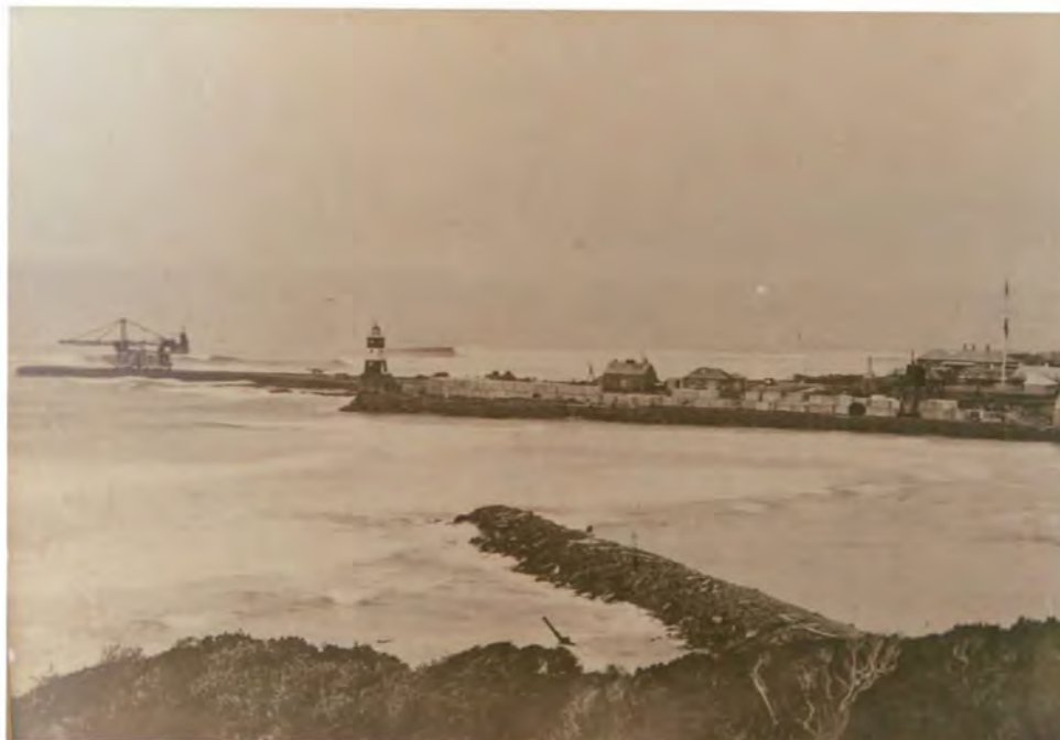
EARLY STAGES IN THE CONSTRUCTION OF THE HARBOUR (about 1876): The eastern training wall (closest) has been partially constructed and the Goliath crane can be seen laying concrete blocks on the southern breakwater. Note that the river mouth is still so shallow as to be only about knee-deep. [ Source: East London Museum.]
