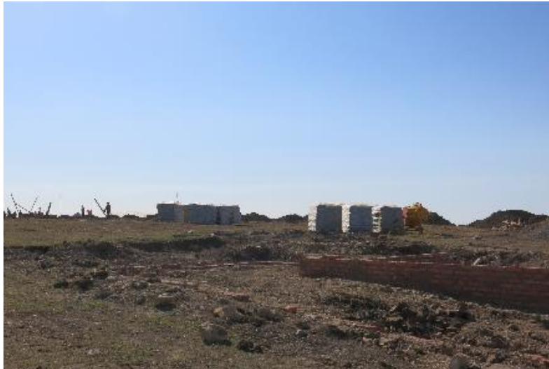
Figure 18: Construction of the Nkonkwana Junior Secondary School underway without electricity or water services (October 2014).
