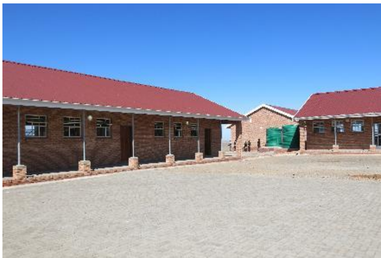
Figure 10: Three newly constructed classroom blocks at Kunene Junior Secondary School.
