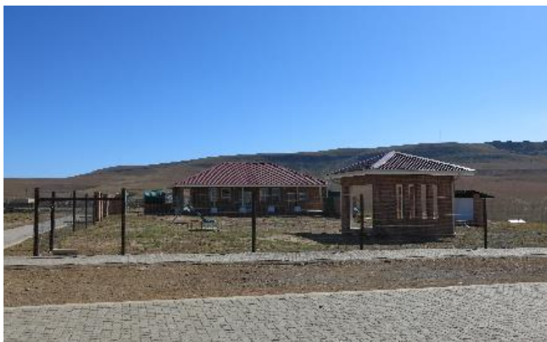
Figure 11: The newly constructed Grade R area at Kunene Junior Secondary School.
