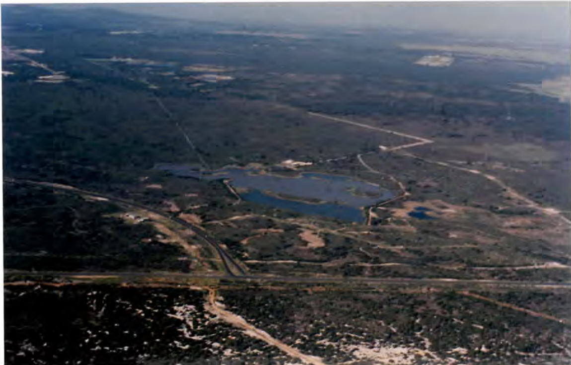
PLATE 6 The artificial recharge basin as seen from the coast with Witzand well field in the foreground and Atlantis township and sewage works in the background (upper left corner).
