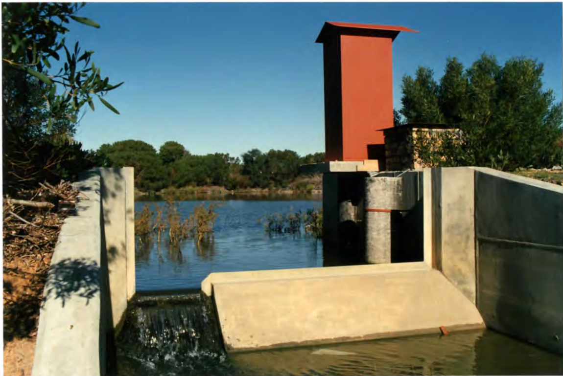
Plate 5 The flow gauging station situated between the stilling pond and the main retention basin (Pond 7)
