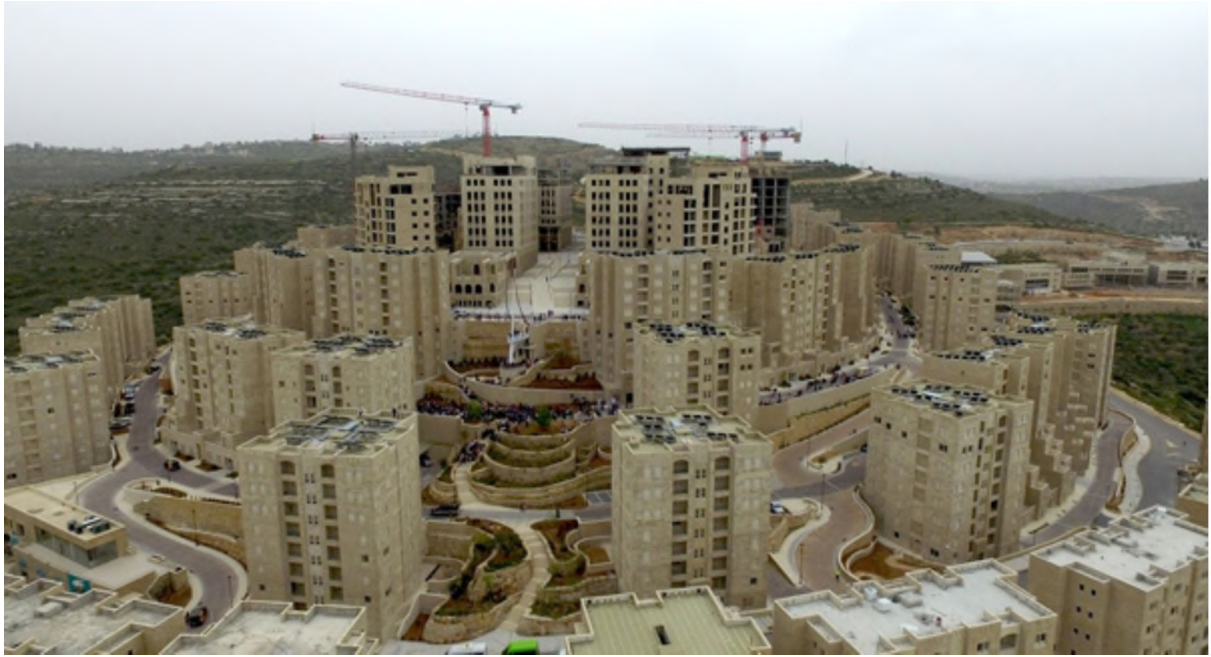
Figure 3.34: Photographic documentation of the Rawabi settlement currently under construction, 2016 (www.rawabi.ps 2016).
