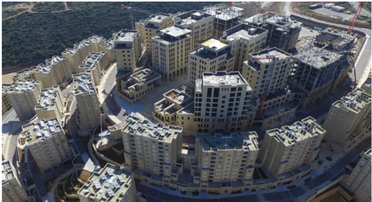
Figure 3.41: Photographic documentation of the Rawabi settlement currently under construction. (www.rawabi.ps 2016).
