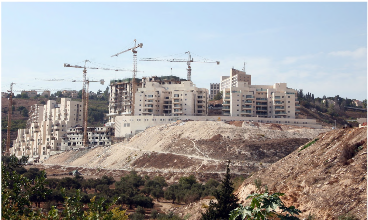
Figure 3.39: Photographic documentation of illegal settlement construction in the West Bank (www.rawabi.ps 2016).
