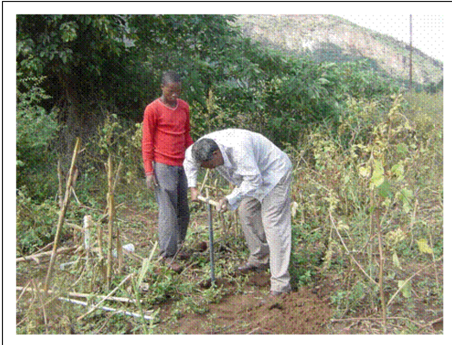
Figure 4.3 Augering for piezometer installation at Kudumela Wetland, Limpopo Province
