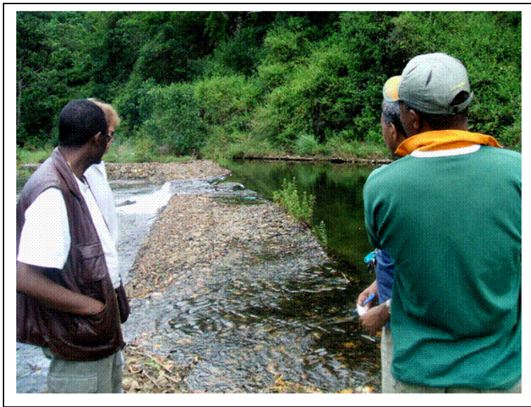
Figure 2.3 Gabion dam structure at the head of the valley
