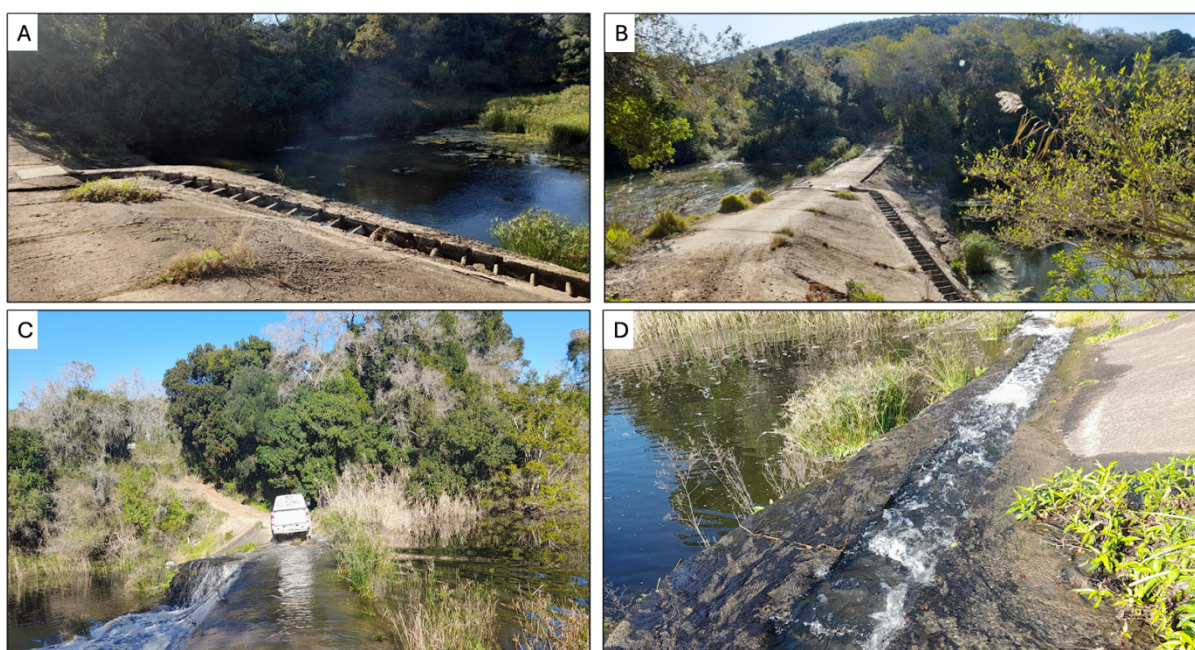
Figure 2.7. The Kowie Weir and fish ladder during (A and B) low flow on the 7 th July 2022 and (C and D) high flow on the 2 August 2023.
