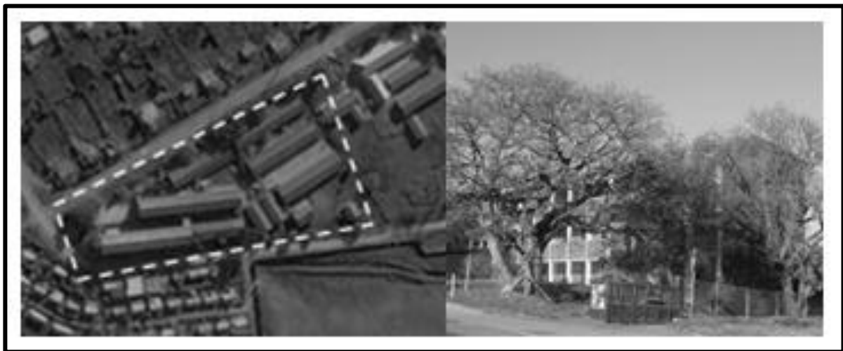
Figure 5.14: Nathaniel Nyaluza's Facilities (Source: Google Earth, 2003)
