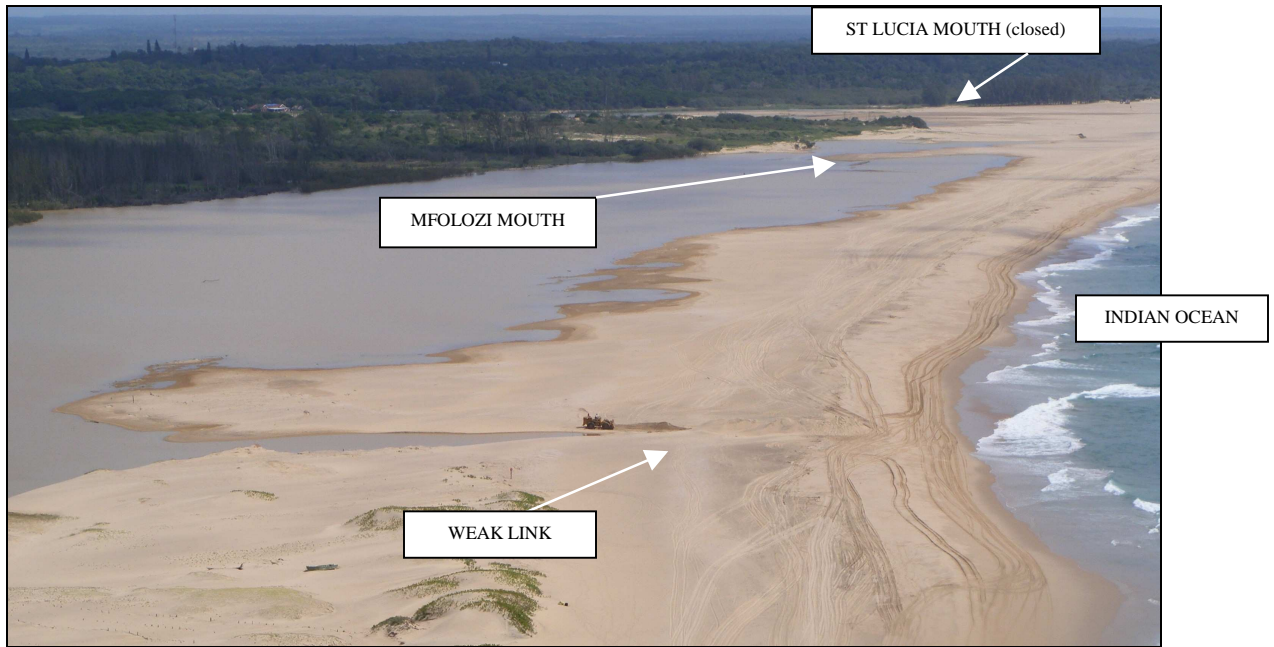
Figure 10: A bulldozer constructing a 'weak link' to prevent the northwards migration of the Mfolozi River. (Terminology of Whitfield and Taylor, 2009; Photo: S. Collings, November 2008).
