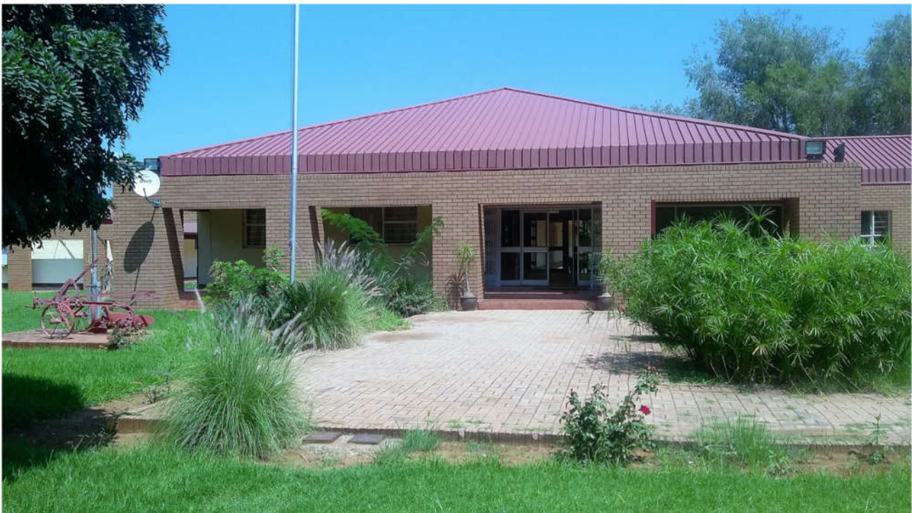
Figure 4.2: The entrance to the main building and lecturing facilities at Taung Agricultural College
