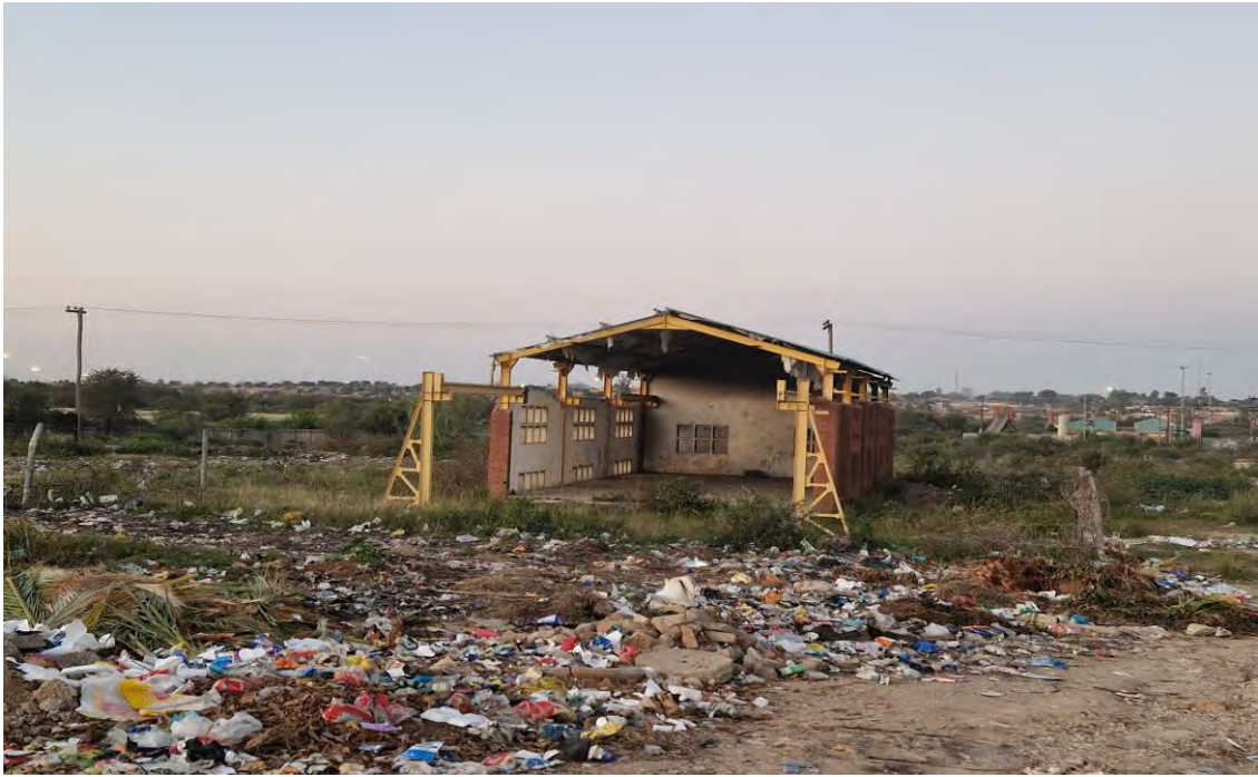
Figure 5.8: Pollution and vandalism at the Leeuwkraal Dam wastewater treatment facility
