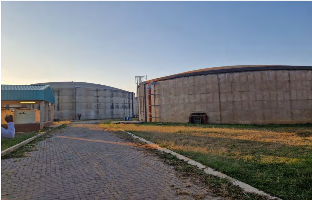
Figure 5.2: Reservoirs at the Temba Water Purification Plant
