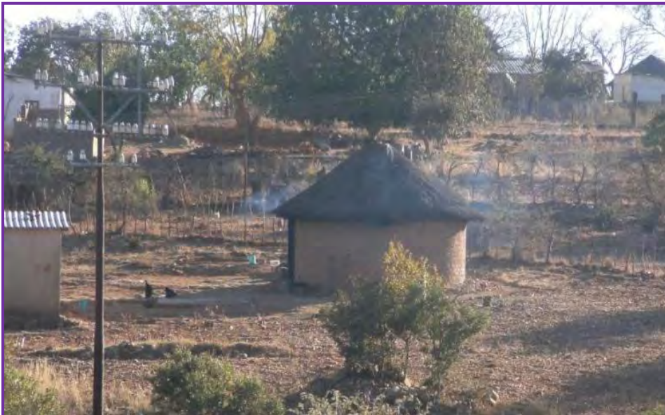
Figure 55: A contemporary Ndebele rondavel with entrance facing west, just before reaching Gwanda Town along the Beit Bridge - Bulawayo road. Matebeleland South, Zimbabwe.
