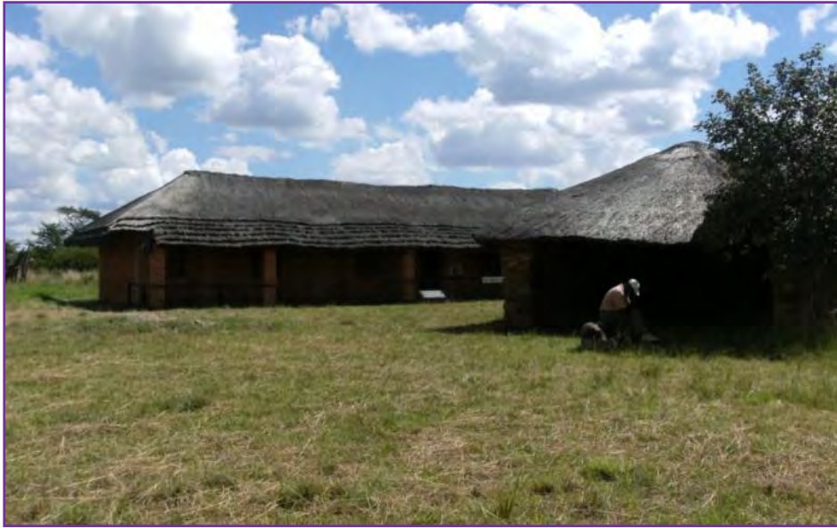
Figure 52: NMMZ. King Lobengula's house in brick and thatch (L) and his wagon shed in stone and thatch (R). Old Bulawayo, Zimbabwe. [15 April 2010]
