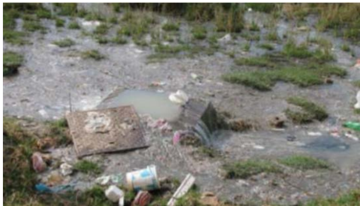
Figure 7.1 Untreated wastewater overflowing from a manhole into the uMthinzima Stream, Mpophomeni (Source: Ward, 2016)
