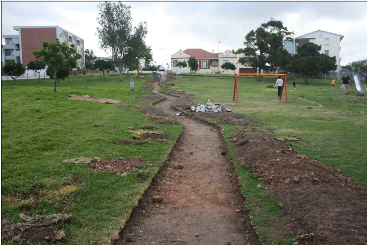
Figure 26 The unauthorised work being done in the Old African Burial Ground/Richmond Hill Park. Photograph by author, 19 November 2023.
