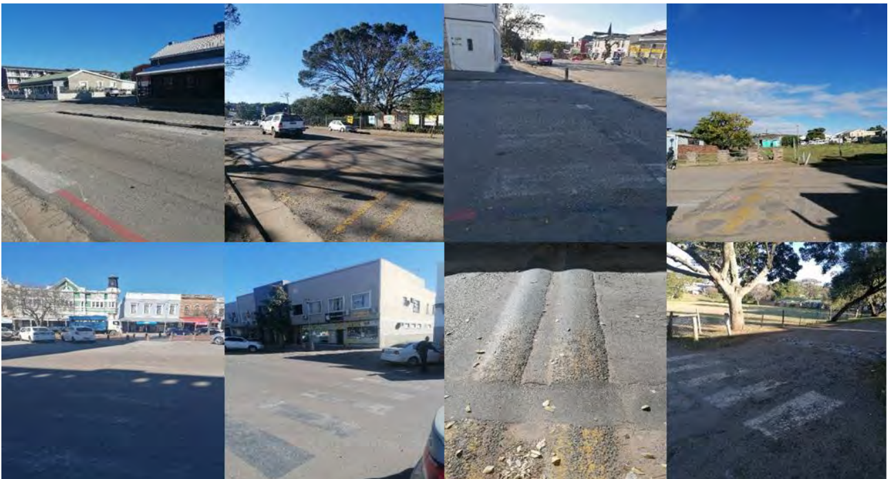
Figure 5.4.3c. An illustration showing poor visibility of markings within the four study areas.
