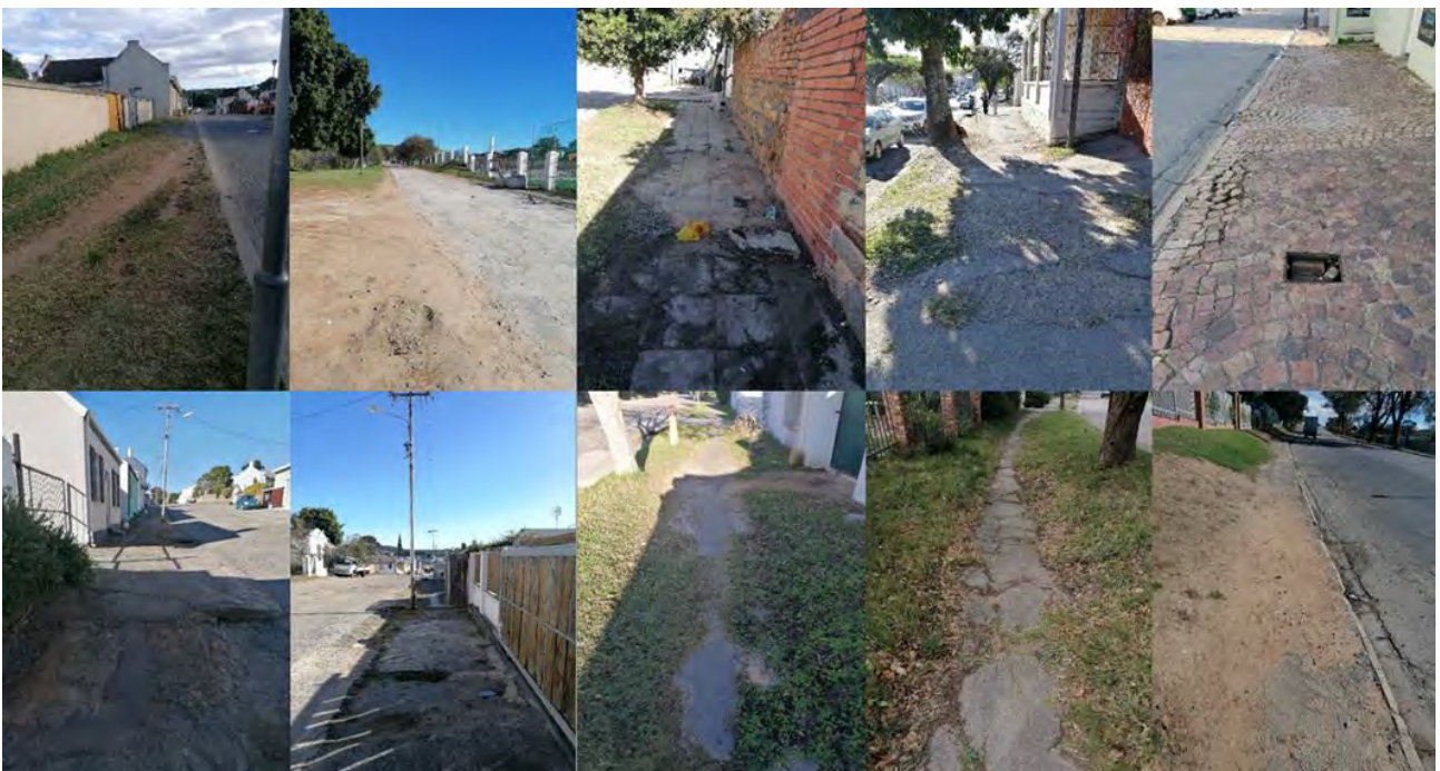
Figure 5.3.7b. An illustration showing fair sidewalk condition within the four study areas.
