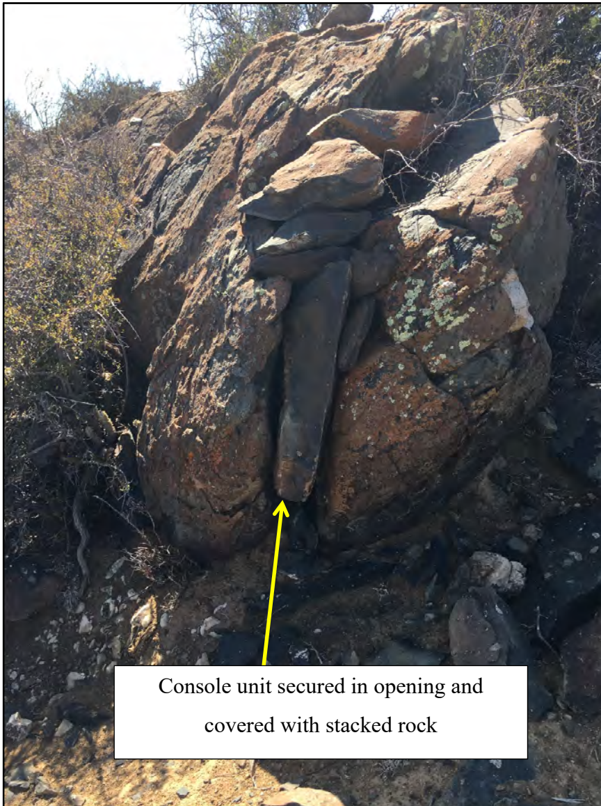
Figure 3.7: Weather station console enclosure
