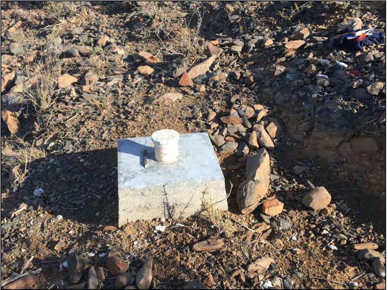
Figure 3.1: Block and standpipe capping used to seal borehole shafts
