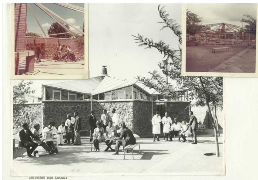
Fig 5.9 Images of Chiweshe bar under construction and outdoor scene
