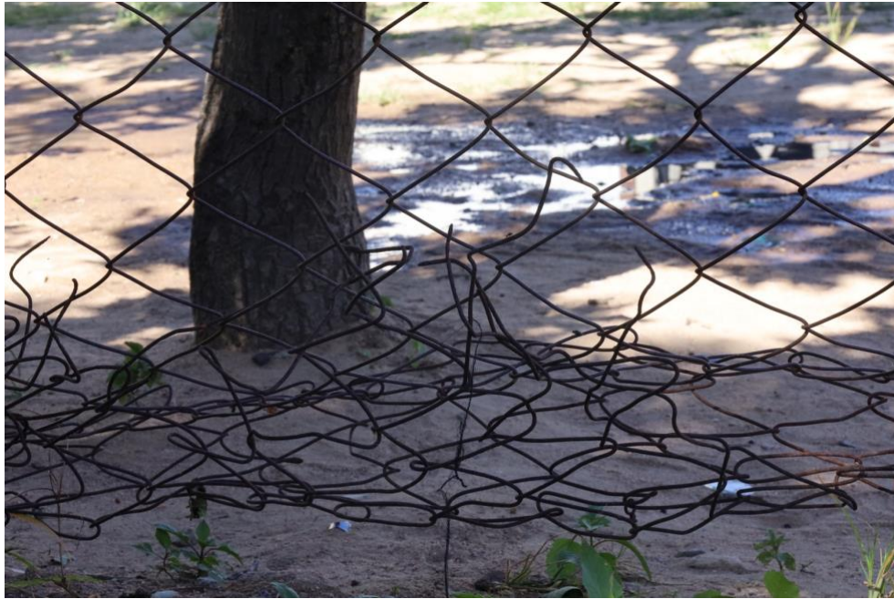
Fig 3.5 The old wire fencing at Johnson Zuze's neighbourhood, Chitungwiza, Harare, 2021.
