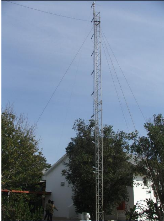
Figure 3.2: The 12 m mast on which the inverted-vee dipole antenna was installed.
