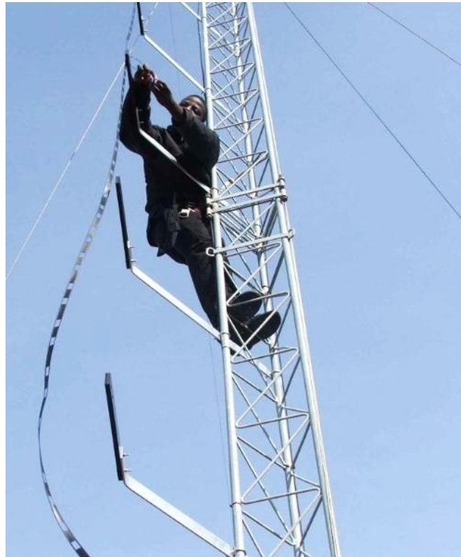
Figure 3.5: G5RV antenna installation on the 12 m mast.
