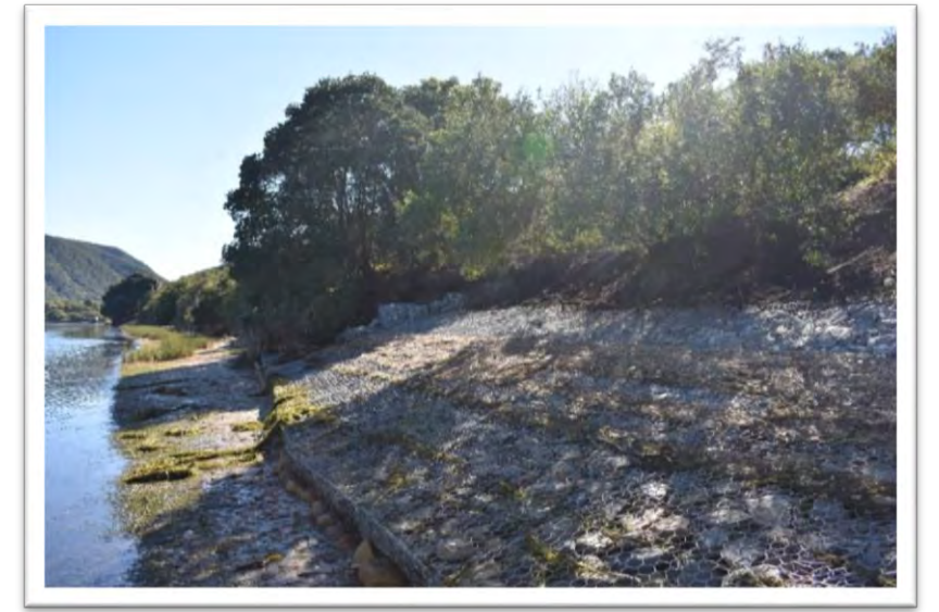
Photographs of the installation of the new erosion control structure Reno-mattress along the eastern bank of Keurbooms Estuary (before installation on the left, after installation on the right).
