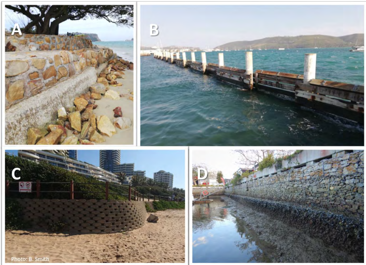
123 124 Figure 1.2. Different types of artificial structures commonly used in erosion control along coastlines. 125 A: Sea wall of Leisure isle within the Knysna Estuary, B: wooden retaining wall of the Knysna 126 Harbour, C: Loffelstein walls make up part of a promenade in Umhlanga (KZN), D: Gabions form the 127 walls and canals of Thesen Island Marina in Knysna.
