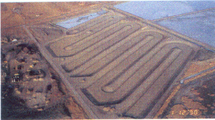
Viet Ngo Devil's Lake Waste Water Treatment Plant 1990
