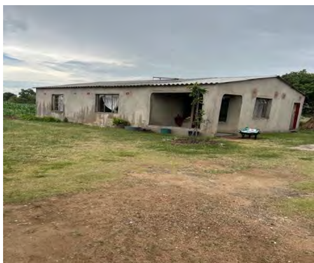
Photo 3: A house in Kanzou Village with a solar panel on top.
