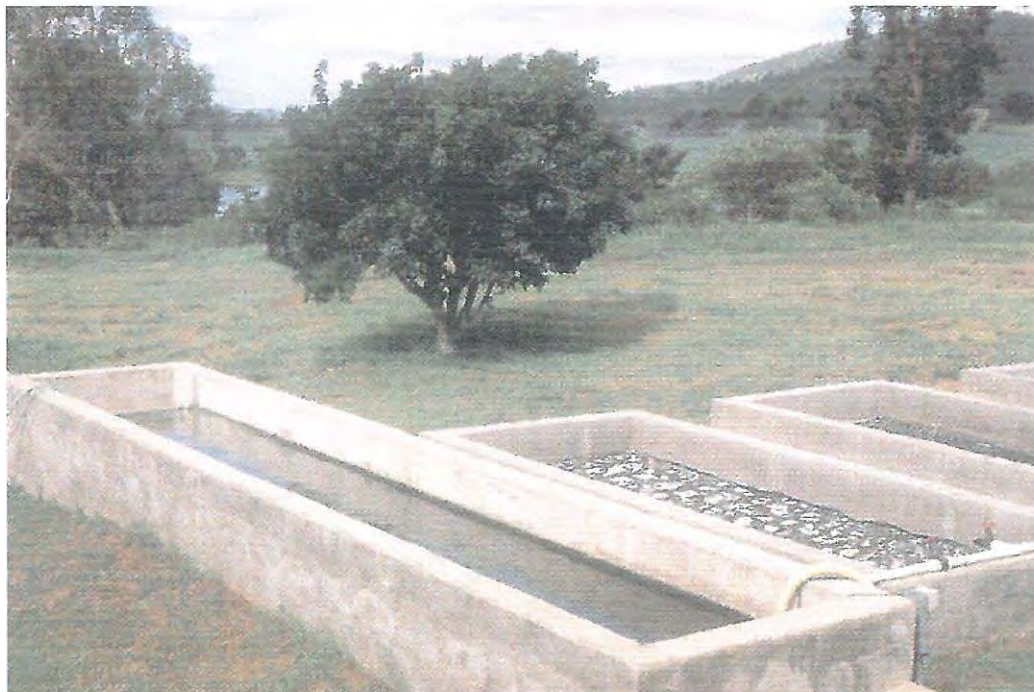
Figure 1.7. Algal settling unit with sand drying bed, Environmental Biotechnology Field Station, Grahamstown.
