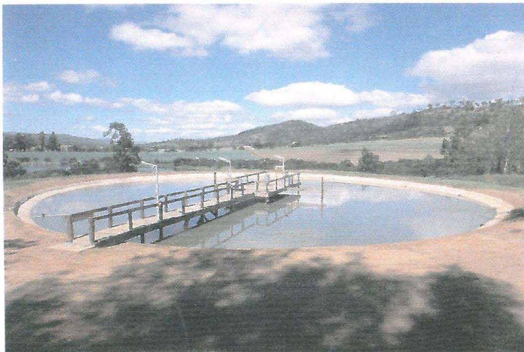
Figure 1.5. The primary facultative pond, Environmental Biotechnology Field Station, Grahamstown.
