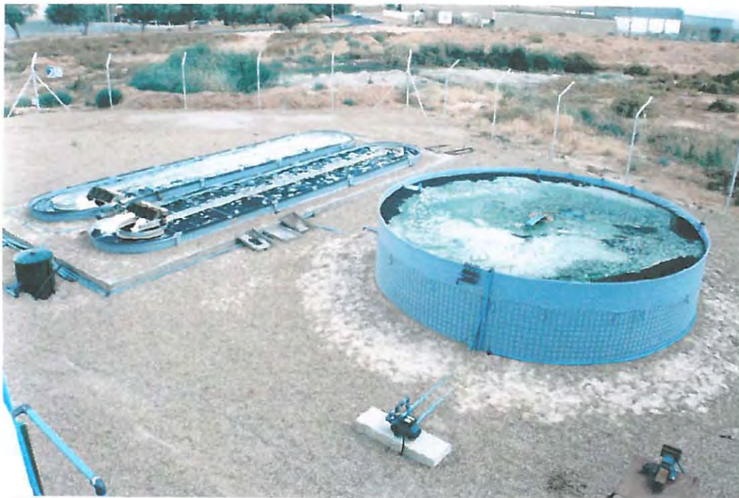
Figure 6.3.3. Photograph of the Integrated Algal Ponding System showing the Facultative Pond (right) and the two High Rate Algal Ponds (left).
