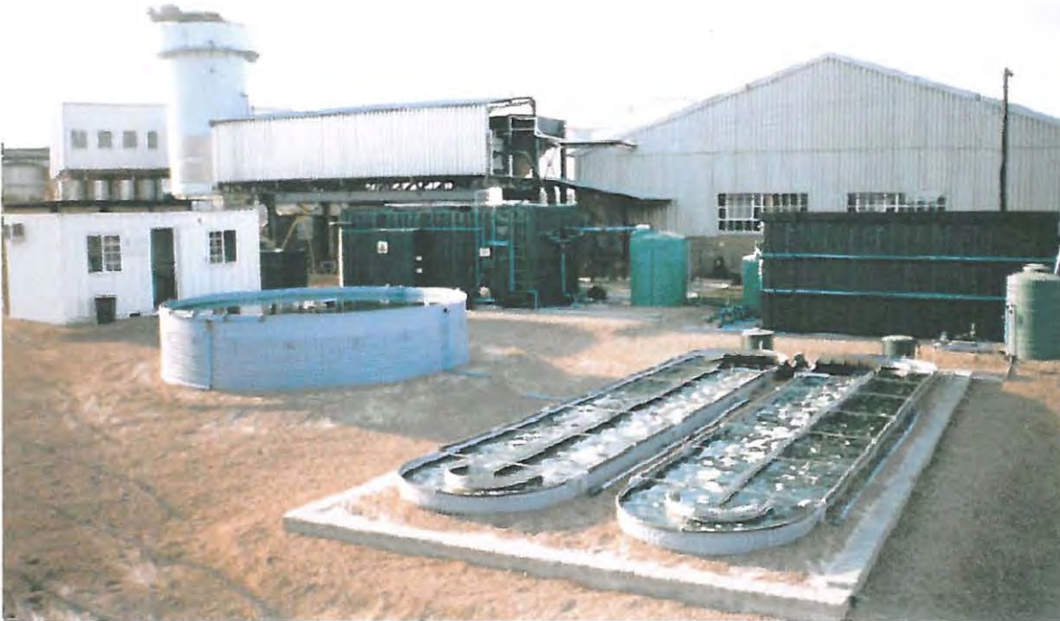
Figure 6.3.2. Photograph of the Rhodes University pilot plant at Brenn-O-Kem, Worcester, showing the Buffer Tank (left rear), the two Anaerobic Baffle Reactors (centre rear & right), the Facultative Pond (centre left) and the High Rate Algal Ponds (front right), and the site laboratory (left).
