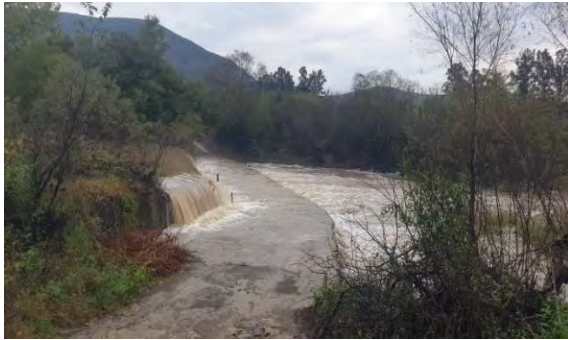
Figure 4.9 Small bridge overflowing during a heavy rainfall in the Kat River catchment
