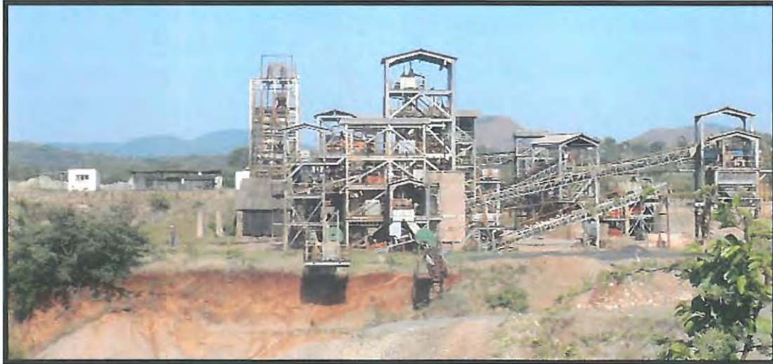
Fig. 1.8 Eluvial Concentrator Plant
