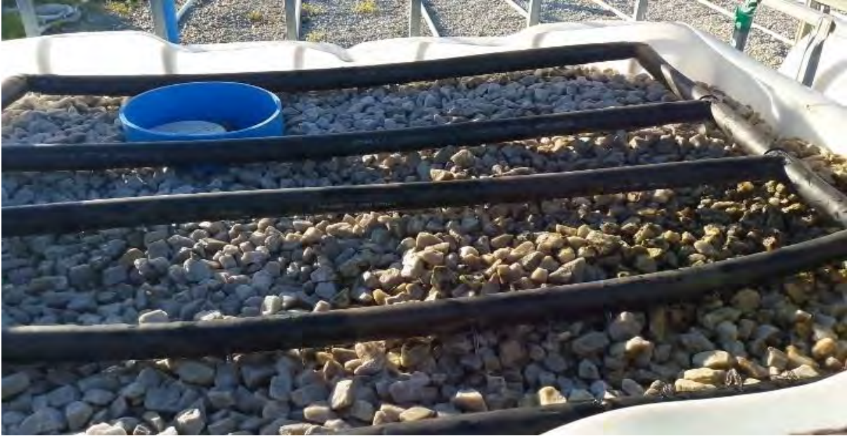
Figure 4.1 The trickle filters were made with 30 mm piping with holes drilled every 7 cm to release steady streams of effluent over the surface of the gravel. The gravel guards (blue piping pictured in the left-hand corner) remained in place from the ebb and flow filters but the bell-siphon and standpipe inside were removed to allow the effluent to exit the filter continuously.
