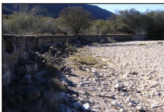
Figure 2.14: Main channel bed and bank erosion on the farm Rus en Vrede, study site 9.
