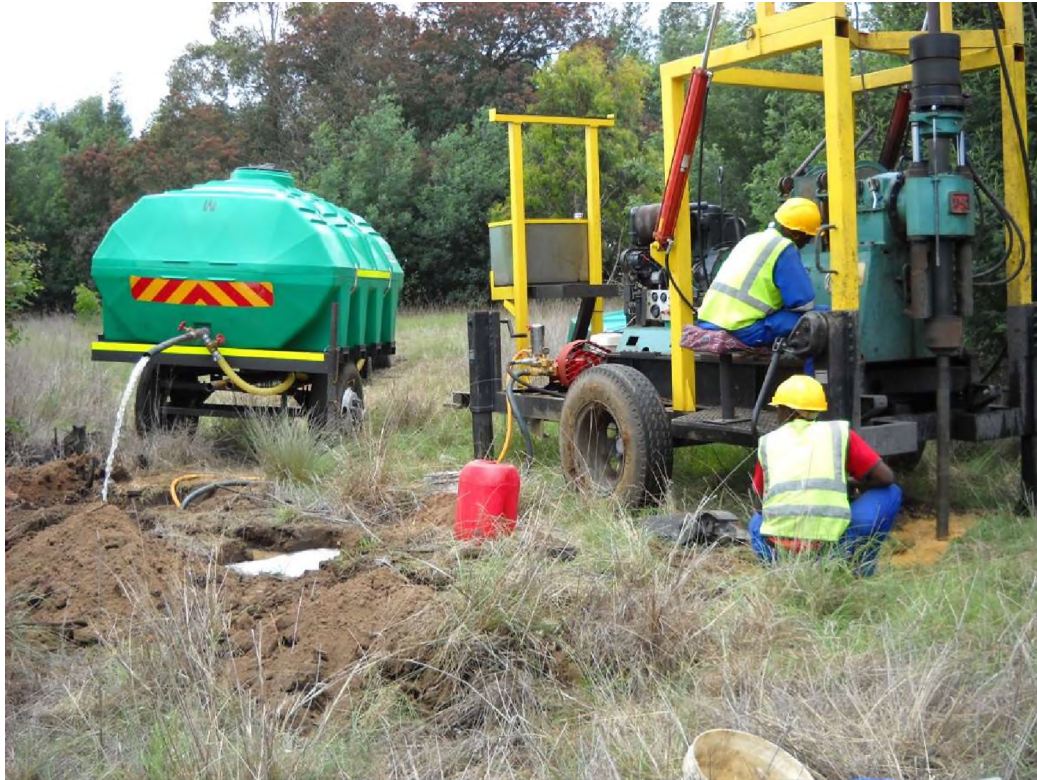
Figure 14. A diamond drill rig in operation.
