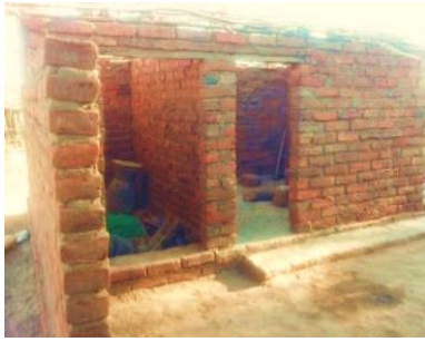
Photo 7.11: Newly constructed kitchen (Chisoni, June 2016b)
