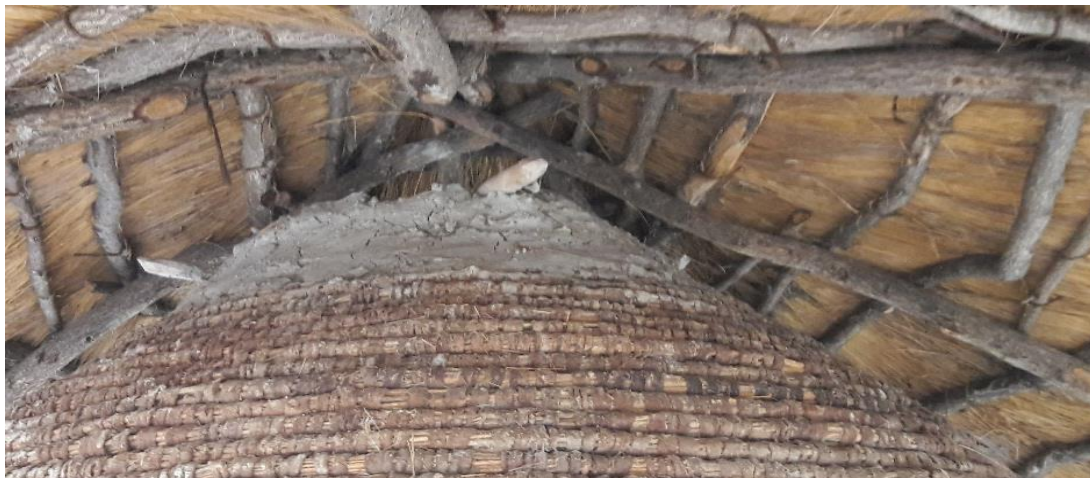
Figure 5.2: The oshimato (lid) plastered over with mud
