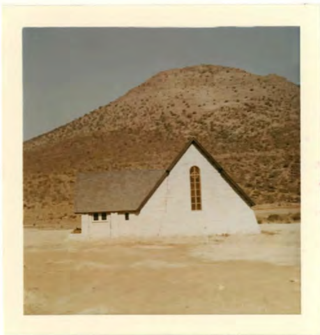
The Presbyterian Church at Eildon, built 1958.
