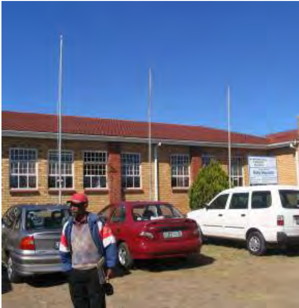
Photograph 70: The façade of the school
