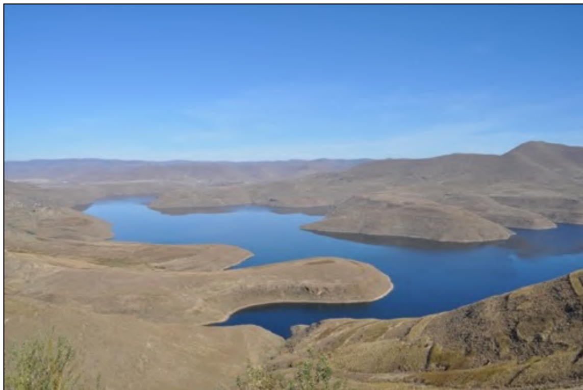
Figure 3.4: Katse Dam is situated on the Malibamatso River and forms part of Phase IA of the Lesotho Highlands Water Project; the dam is characterised by steep rocky and grassy shorelines with a limited littoral zone.
