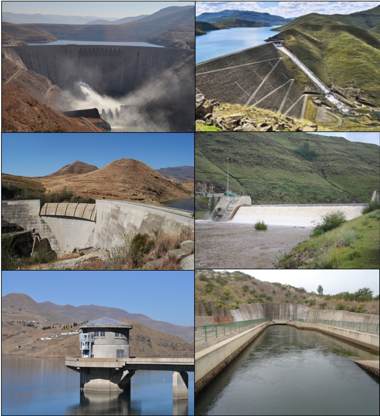
Figure 2.10: Phase I of the Lesotho Highlands Water Project includes the Katse Dam (top left) (Source: Stuart Slabbert); the Mohale Dam (top right) (Source: LHDA); the Muela Tailpond Dam (middle left) (Source: LHDA); the Matsoku Weir (middle right) (Source: LHDA); and 140 km of tunnels (bottom left and bottom right) (Source: Beniamino Pellegrini) that deliver water from the Lesotho Highlands to South Africa.
