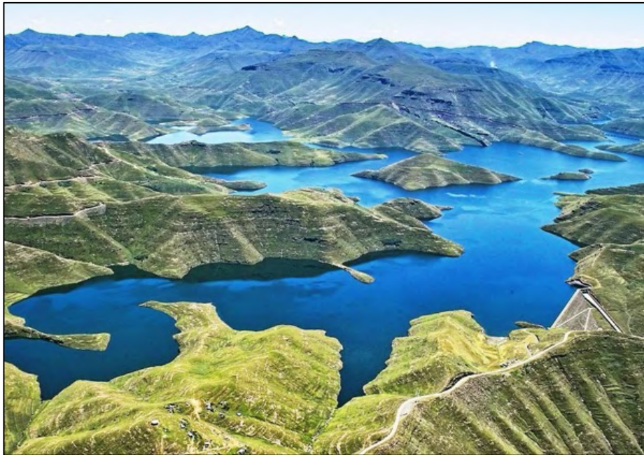
Figure 6.2: Mohale Dam is situated on the upper Senqunyane River catchment and forms part of Phase IB of the Lesotho Highlands Water Project (Source: Stuart Slabbert 2012).
