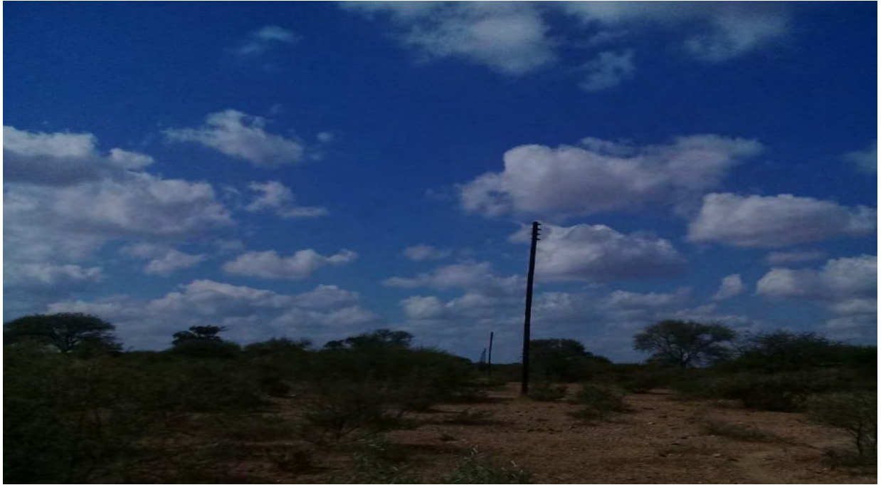
Fig 5. Electricity pylons navigating their way through the acacia shrubs in Makhubu. The electricity is one of the few innovations seen in the area for decades. Regrettably it only services a few mines. Locals do access it for simpler tasks like charging cell phone batteries. At its current cost it is safe to say that most of the locals would not be able to purchase it for domestic use.
