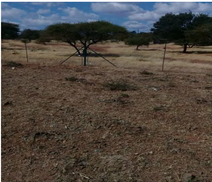
Figure 6. The picture above shows the electrified fence of the Mphakathi stamping mill, Makhubu.
