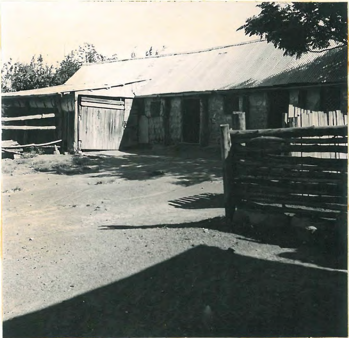
Outbuildings of a German farmstead at Frankfort. The sod walls are part of the original dwelling house. The galvanized iron roof is relatively new and the garage is a recent addition. A corner of the cattle kraal in right foreground.
