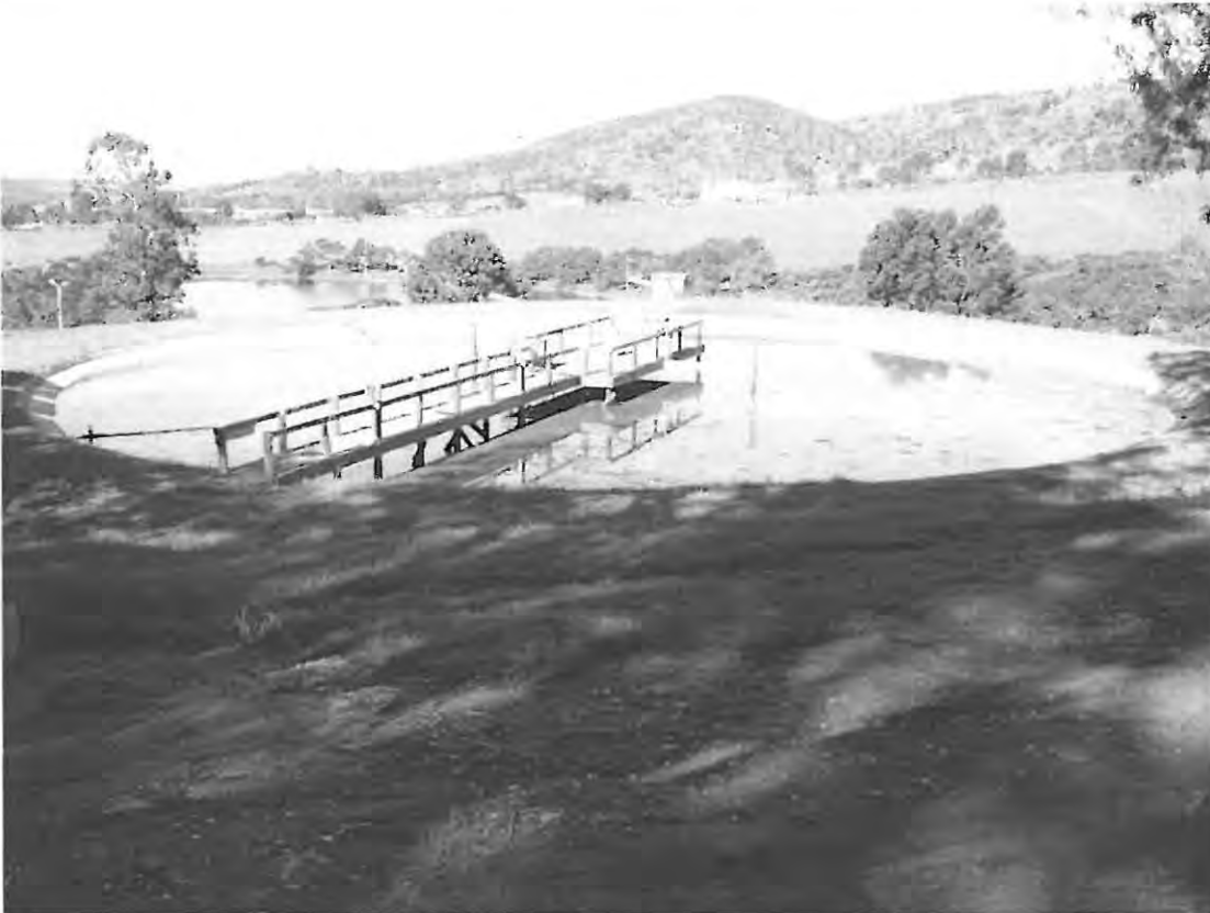
Figure 2.2 The Primary Facultative Pond at the Algal Integrated Wastewater Ponding System pilot plant in Grahamstown, South Africa. The wooden walkway was constructed for experimental access. The Fermentation Pit is submerged below the surface of the PFP at the centre of the pond.
