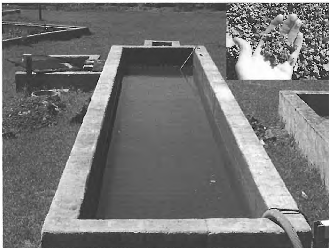
Figure 2.5 A basic algal settling pond as used in the IAPS pilot plant at Grahamstown, South Africa. The insert shows the appearance of dried algae after being pumped from the algal settling pond into the algal drying beds.
