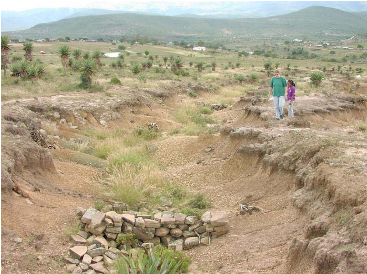
Plate 6.1 Landcare rock structures at an eroded gully in Fairbairn (Photograph supplied by Kate Rowntree)
