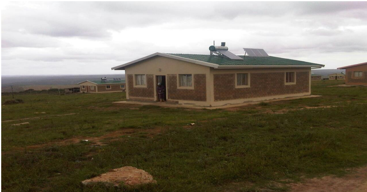
Fig 4.4.: Houses built for the evicted farmworkers by the DRDLR fitted with solar power, water harvesting tanks, and a waste management system at Radway Green Farm as beneficiaries of the land reform programme. (Picture courtesy of the researcher)
