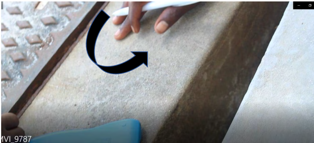
Figure 4.15: L5O spreads her hands to point out the concrete top of the sewage dam
