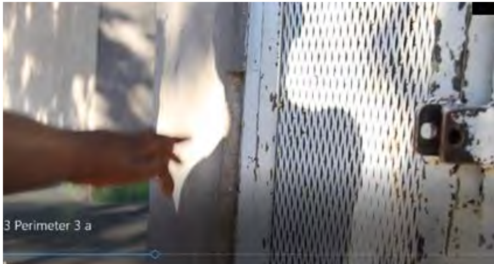
Figure 4. 6: L1O waves at the mesh of the gas cylinder storage
