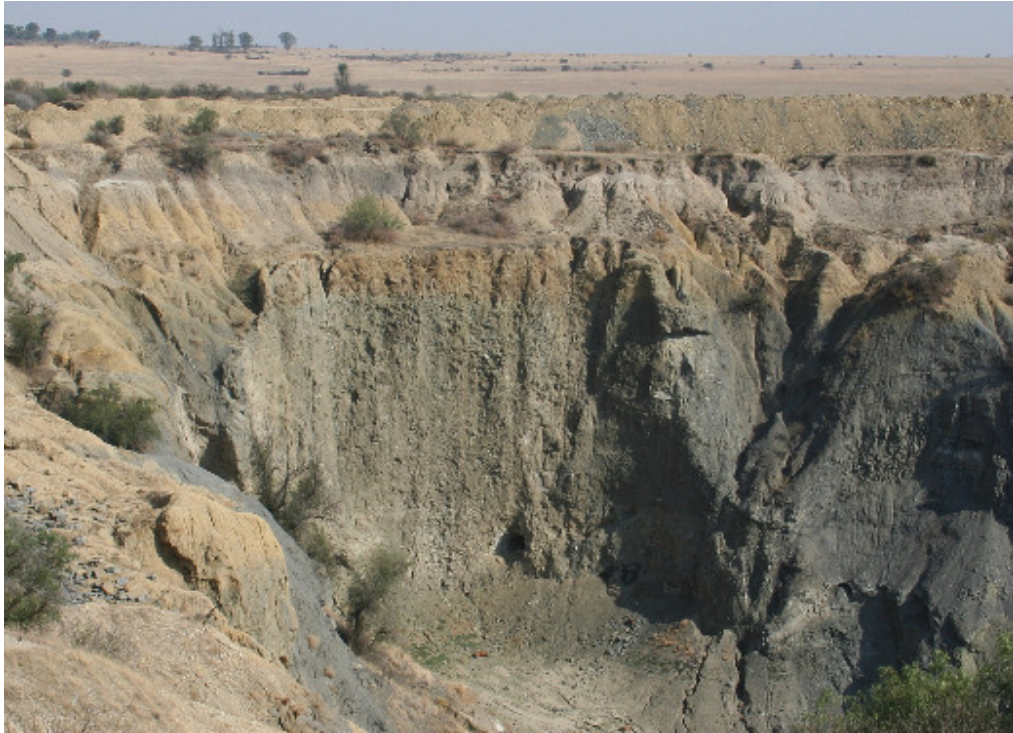
Figure 3.1 Photograph of the Lace pit looking west. The competent rock in the wall is the satellite pipe outcropping in the pit. The pit has been open for over a hundred years and yet no caving of the satellite pipe has occurred indicating the highly competent nature.
